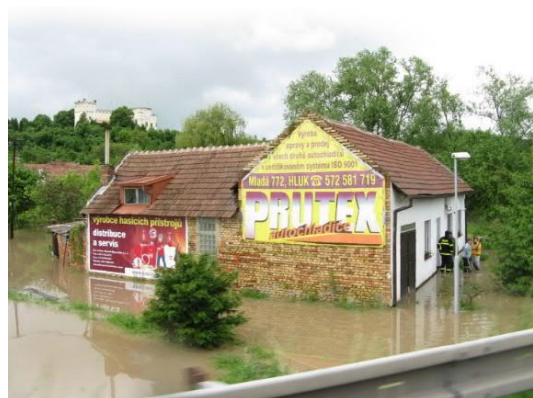
Obr. 2.5 Km cca 42,100 -42,300 LB inundace zaplavenac
