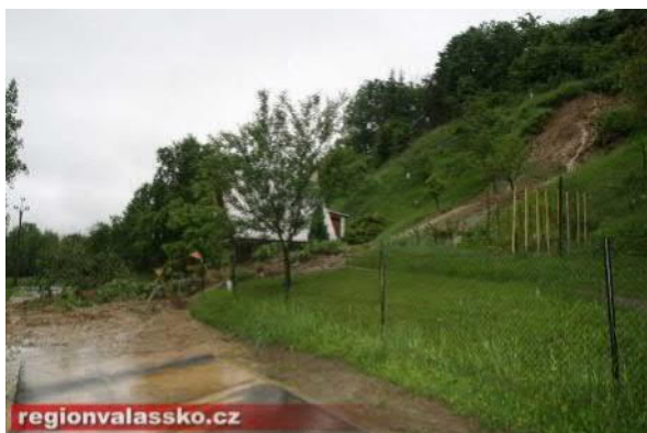
Obr. 2.7 Povodeň 2010 – Brumov-Bylnice, sesuv
